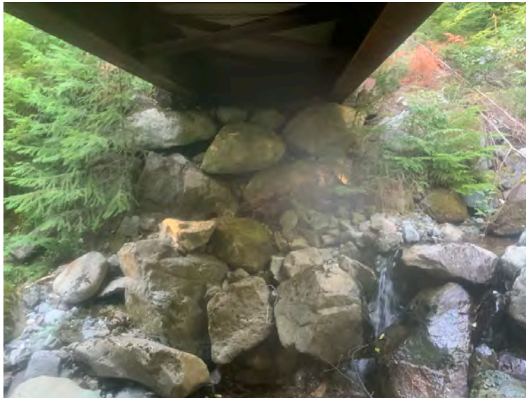
Right Bank Abutment when facing downstream
