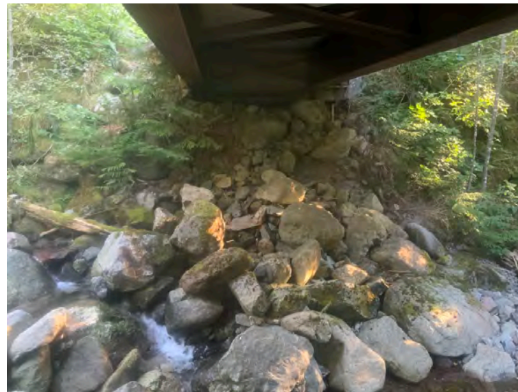
Left Bank Abutment when facing downstream
