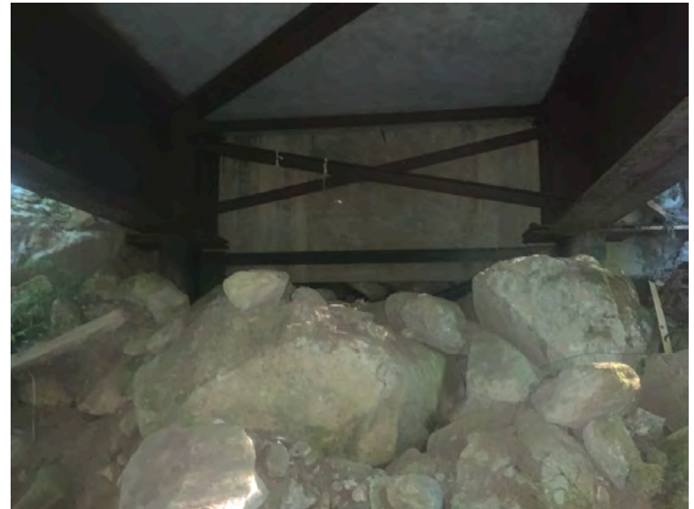
Left Bank Abutment when facing downstream
