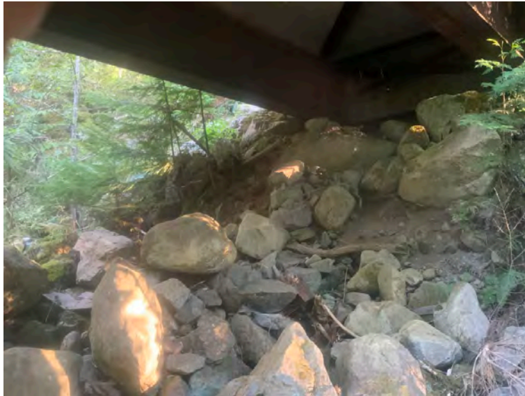
Left Bank Abutment when facing downstream
