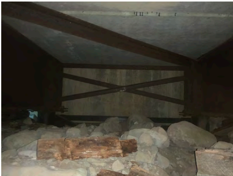
Right Bank Abutment when facing downstream
